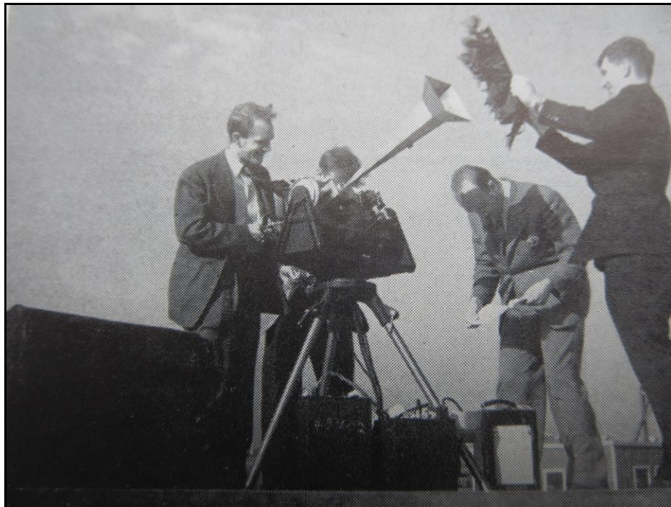
Figure 38- Tipping curve absorption measurements made in 1946 by Dr. Robert Dicke along with his associates. Starting on the Left is E. Beringer, R. Kyhl, A. Vane and R. Dicke. This picture is contained in the MIT Rad Lab Book "Five Years". It shows Dicke holding up an absorber in front of one of his radiometers while a chart recorder on the ground plots the measurements.
